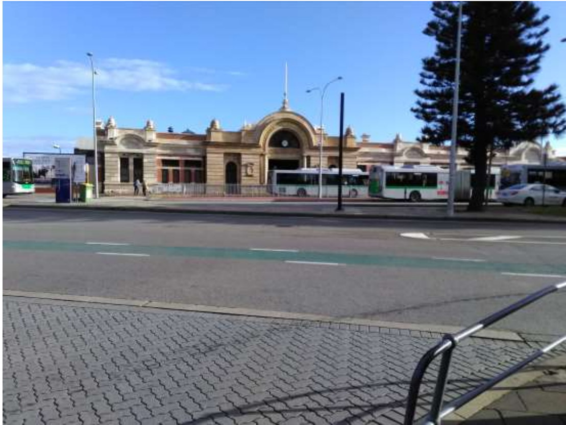
Fremantle Railway Station
